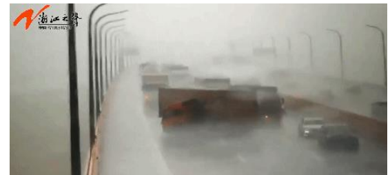
Hangzhou Bay Bridge
