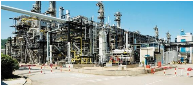
Tai Po Plant
